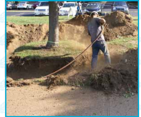
Pneumatic Excavation of heavily compacted soil to aid in the digging.
